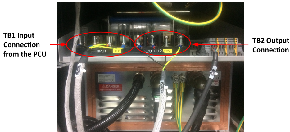
Figure 4.5: HV Output Connections
