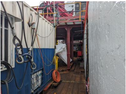
Goose neck on backside of the container for all connections.
